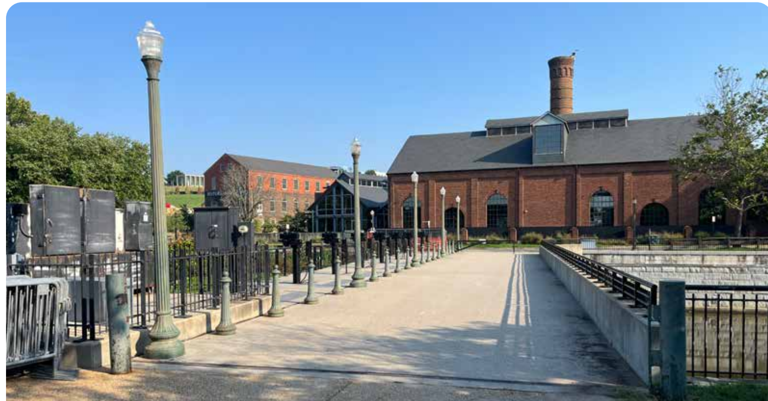
HAXALL BRIDGE LOOKING TOWARDS TREDEGAR
