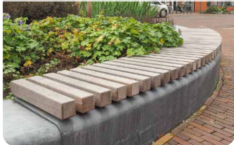
WOOD CLADDING ON SEAT WALL
